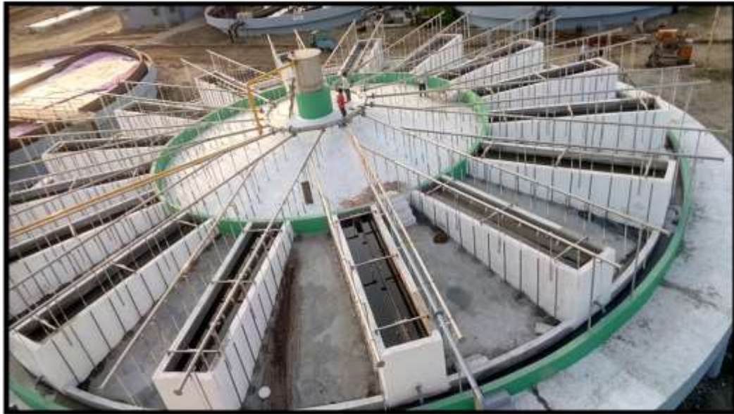
UASB reactor at NEPL (Naroda Enviro projects ltd) GIDC, Naroda Ahmedabad
